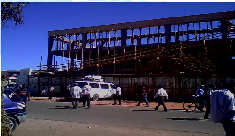
Figure 4: Limited Use of Mechanical Plant
